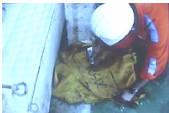
Photo 08 – Preparing the test , only PVC and sail cloth protection
